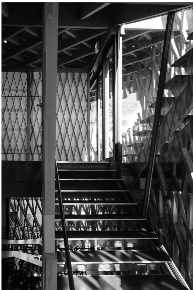
Figure 9. Entrance at Sunny Hills shop by Kengo Kuma in Tokyo. A visitor to the shop pass through layers of wood lattices before entering through the glass doors, then move through additional layers of wood and paper screens once inside. Photograph: Author.
